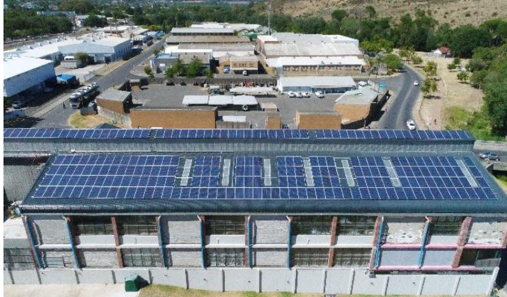
Factory, Western Cape, SA 60 kWp (2018)
