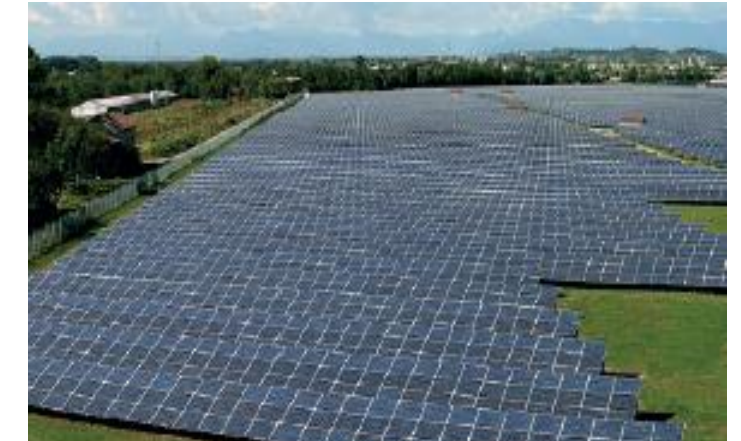
Manzano, Italy 11.2 Mwp (2011)
