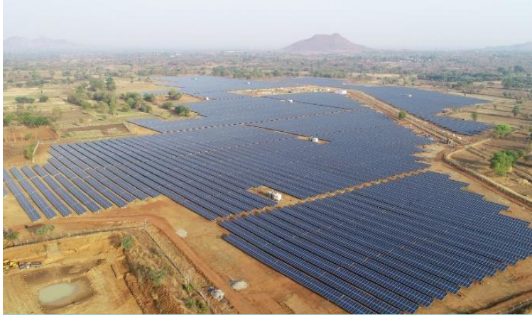
Sadipali, India, 27.35 MWp (2018)
